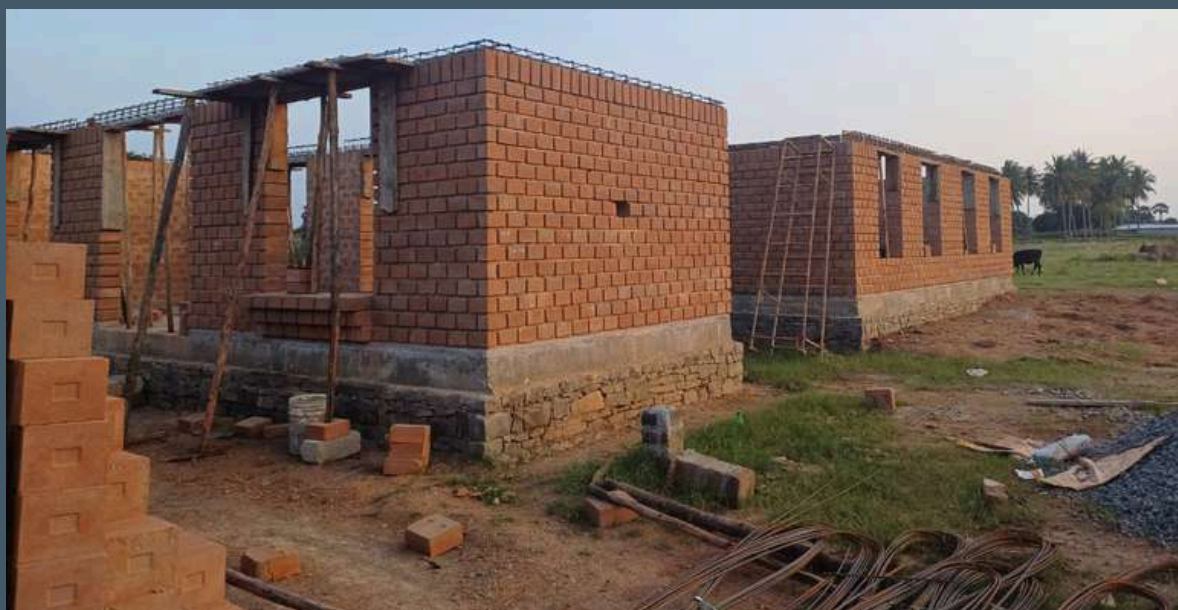
Top: Wellness Centre | Below: Vilvam Learning Center construction work in progress
